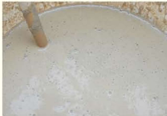
Use this paste to fill the holes and indentations in the brickwork and mortar lines Scrape flush with the surface and leave to dry overnight
