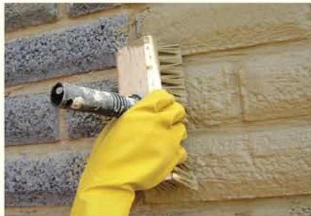
Make sure to fill small holes and indentations
