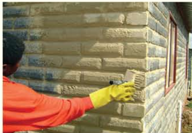
Coat the entire wall in one operation to avoid dry joints Do not stop and start. Do not patch
