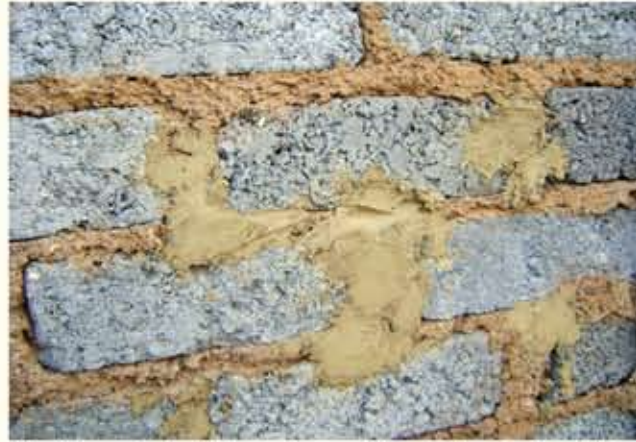
Use this paste to fill the holes and indentations in the brickwork and mortar lines Scrape flush with the surface and leave to dry overnight
