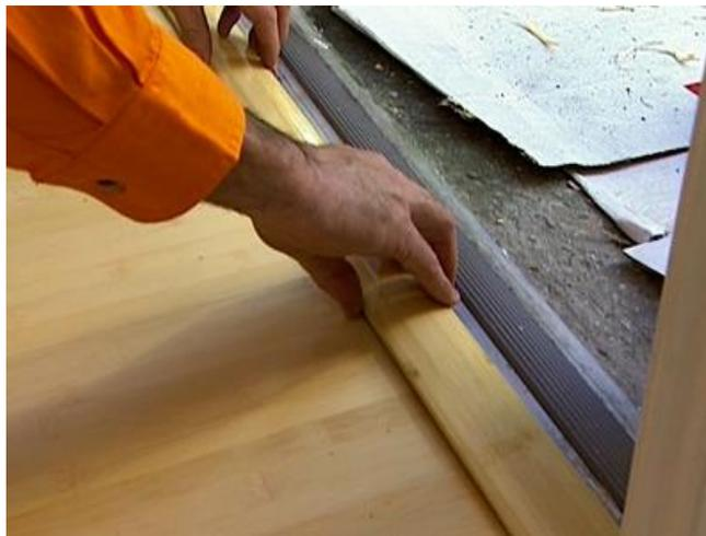
Some Laminate floor types needed to be glued together, always apply a generous amount of the adhesive to the groove and slide the tongue into it. Wipe away all excess glue before it.
